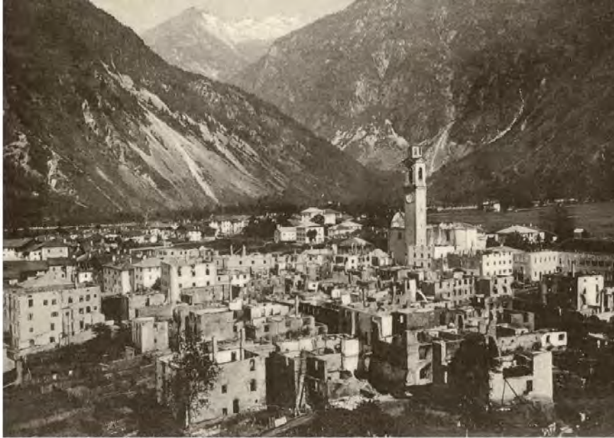
Pinzolo, 27 June 1913; 70 houses destroyed, 135 families homeless
